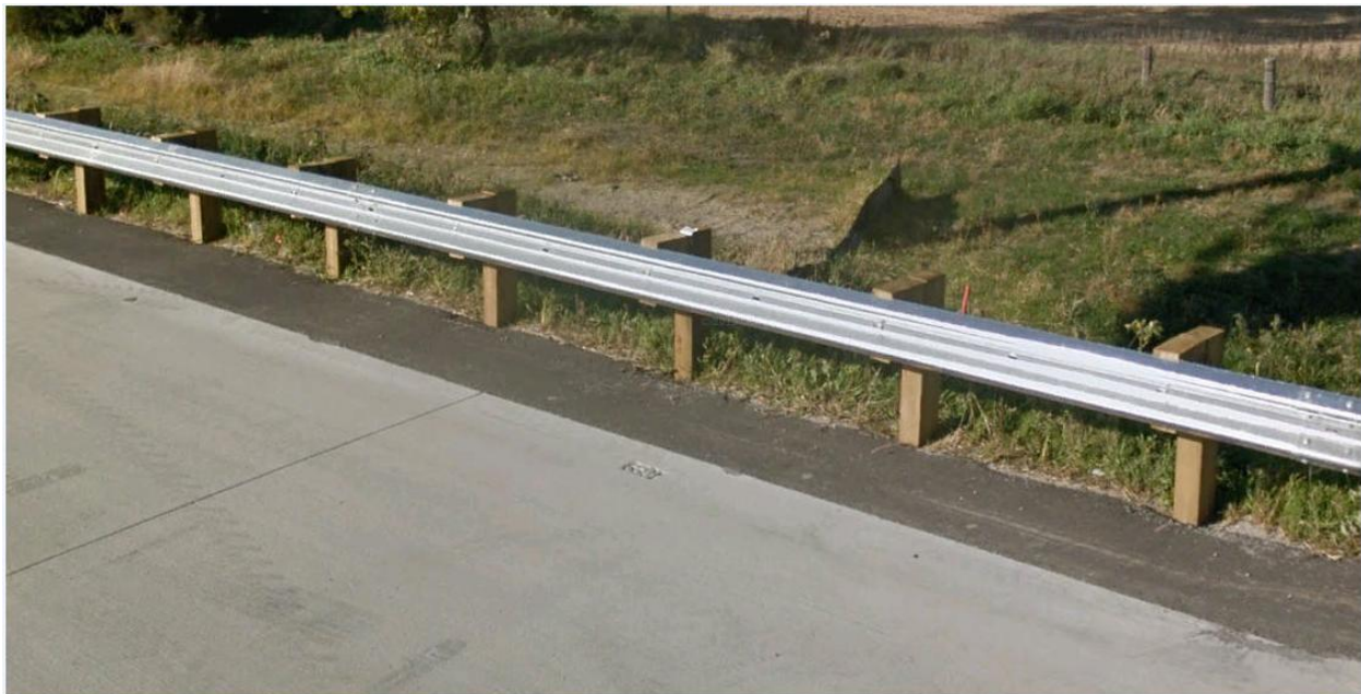
Figure 1: Steel beam guardrail.
