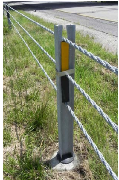
High tension cable guardrail example
